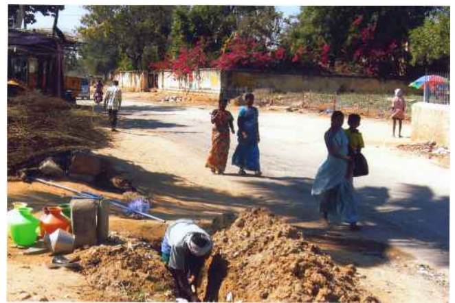
Repairs to Drinking water pipeline leakages
