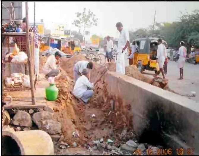
Construction of C C Drain
