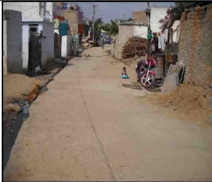
After Complete of the C C Road
